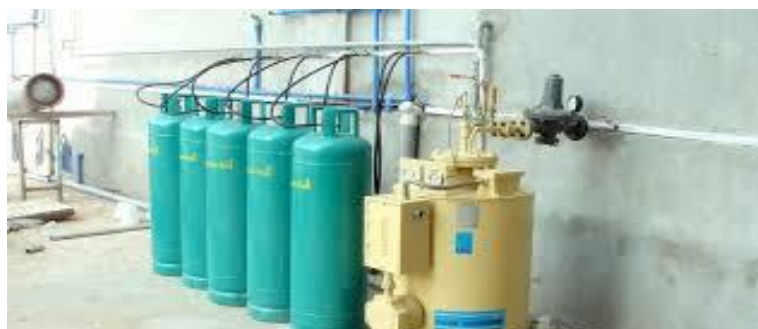
Figure 14: Liquid withdrawal manifold with Vaporizer
