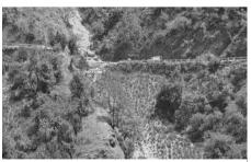
Figure 8: Widening of road lead to erosion of soil
