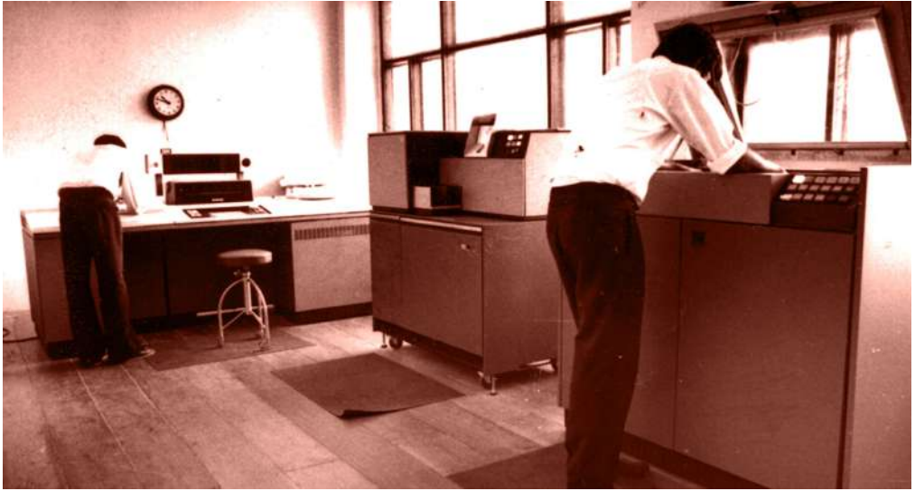
Computer Center of Department of Electrical Engineering in 1975
